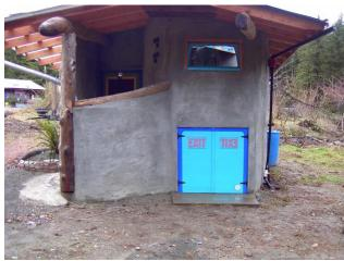
The doors normally are kept fastened with bolts to prevent easy access by children or the public in general. Doors and vents are sealed to prevent fly intrusion.
