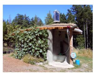
Rainwater from the roof also can be directed into the garden to supplement water supply and also to dilute the salts in the urine.
