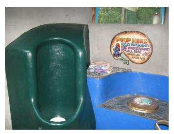
The core function of the building is the recycling of human waste by way of composting. The particular process used is known as vermicomposting, which means using worms to undertake the composting process. The toilet chute leads to a pair of worm bins that are exchanged as required. The organic waste material including paper are digested by the worms and rendered virtually pathogen free. Some of the alder planer shavings, used as a
