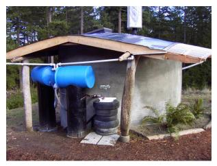
As this water is not for potable use, a torch-on roof membrane was used. Initially both sides of the roof were used for collection until sod was installed on the front half. Water quality was impacted by the soil and so the system was modified so as not to collect from the sod area.
