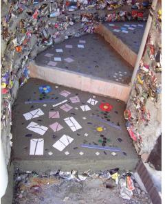
To build up the landings, various "waste" were used such as: broken glass, toaster, vcr's, bricks, small propane bottles, etc., and then a
