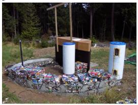
Discarded hot water tanks inside the walls shape the wall ends. These give a pillar effect and visual flow to the structure that nicely complements the spiraling wall. Car windows are used in the wall above the toilet and broken tile and glass are inlaid to various surfaces for finishing touches. Visitors leave with their imaginations inspired by the possibilities presented by building with previously used materials destined for land fill or reprocessing for recycling.
