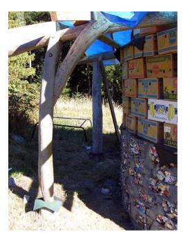
Built like a straw bale post and beam structure the walls of the spiral shaped building are comprised of crushed bales of tin cans, newspaper filled banana boxes, old red bricks, computer printers, toasters, glass bottles, VCR's, etc. Stucco covers all of this giving a finished adobe look. A Plexiglas window shows the inner wall materials.
